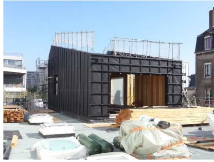
Extension ossature bois
