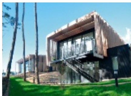
Image 2 Facade de KerGrid
